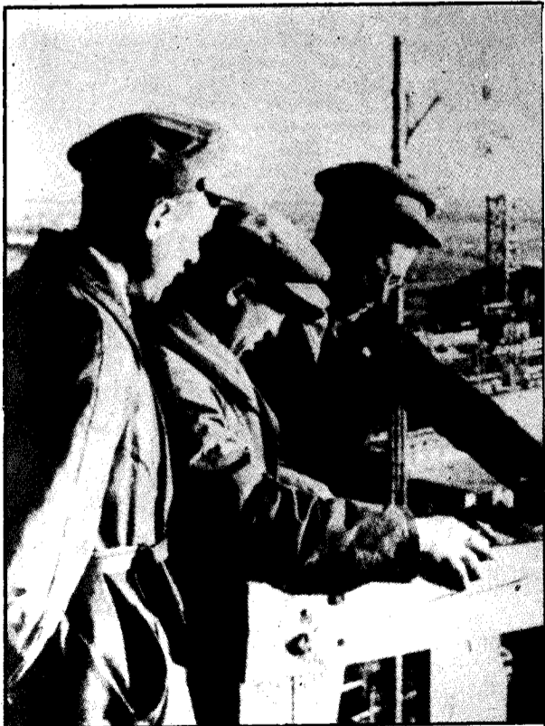
Industrialisation — construction of a coke-chemical plant
